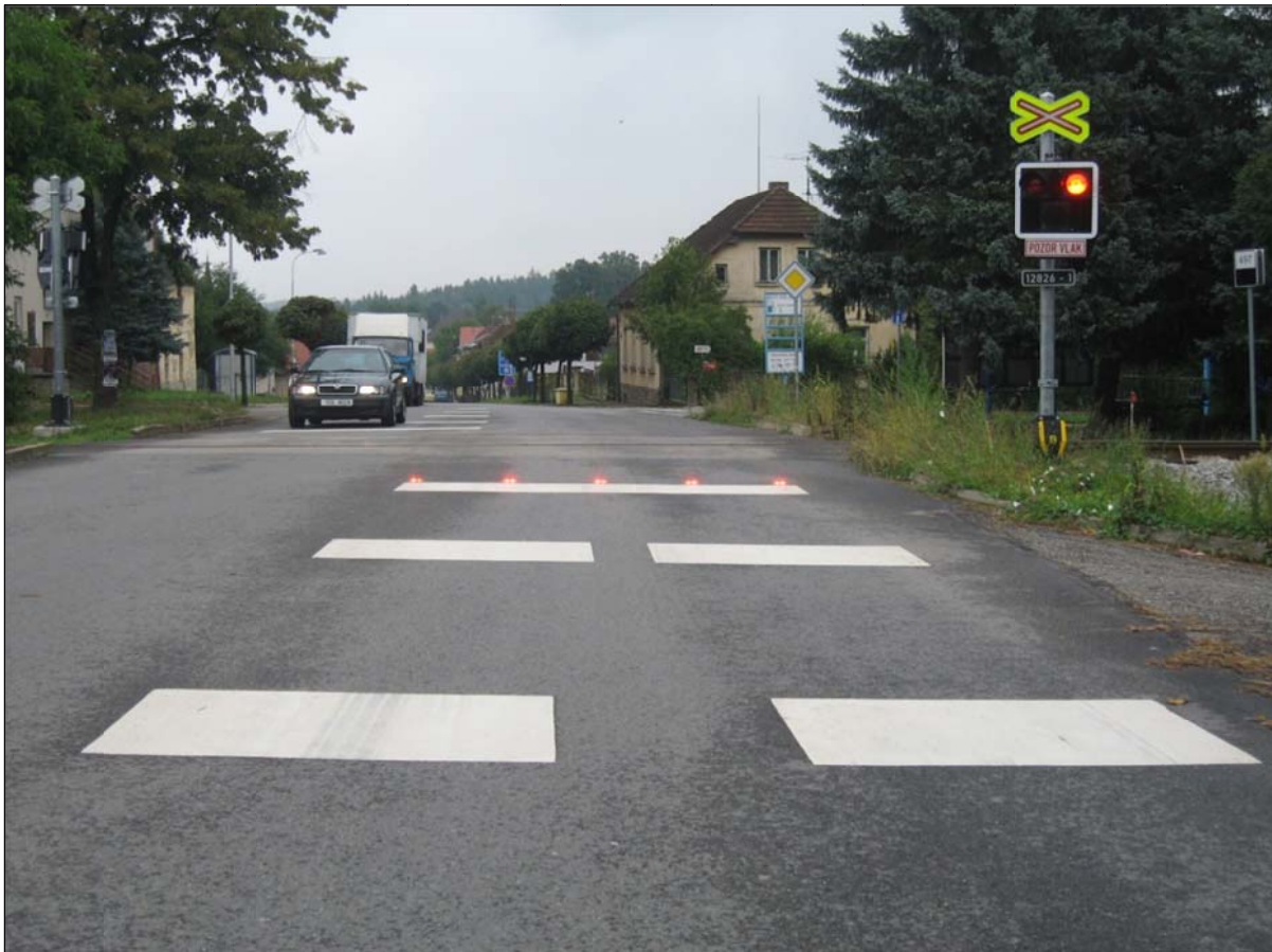
Figure 3. Light barrier and funneled psychological brake in Nová Včelnice
