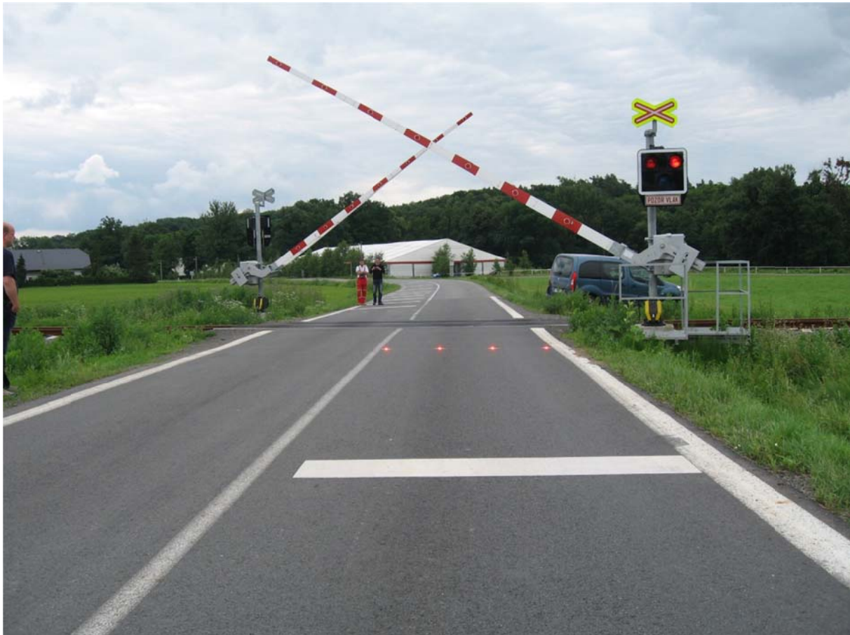
Figure 5. Light barrier combined with additional mechanical barrier in Otice
