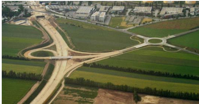
Motorway construction nearby Vienna (© Jan Spousta)
