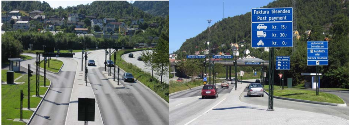
Figure 5: Fully automatic toll stations at Gravdal in the city of Bergen.
