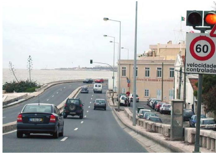
Figure 1 – Speed control with traffic signs (EN 6).
