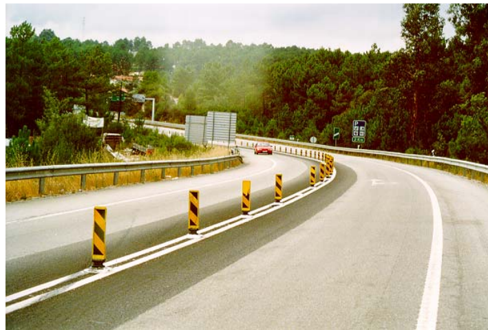
Figure 2 - Application of delineators at the centre line (IP 5).
